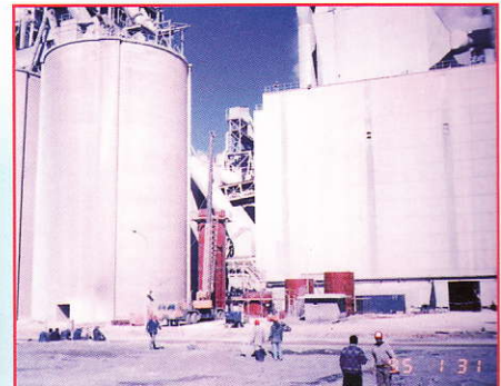
Jordan Cement Plant (FUHES) In Cooperation With F.L. SMITH South Cement Plant
