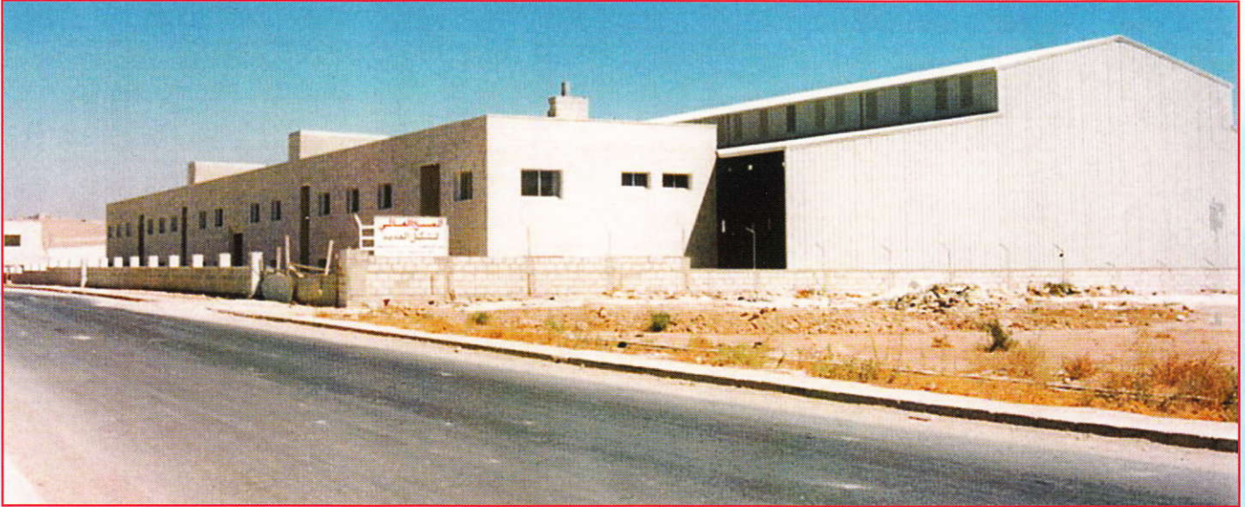
Universal Steel Fabrication Factory ( MEC Factory )
